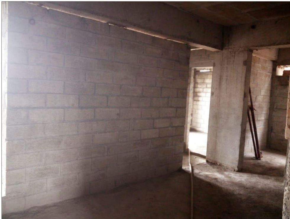
First floor blockwork
