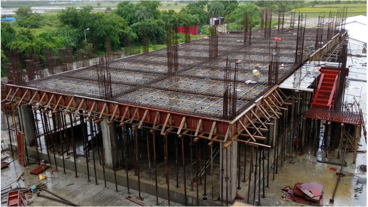
First floor roof shuttering and bar-bending
