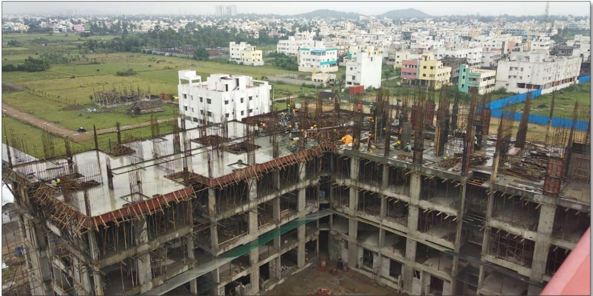
Structure till four floors
