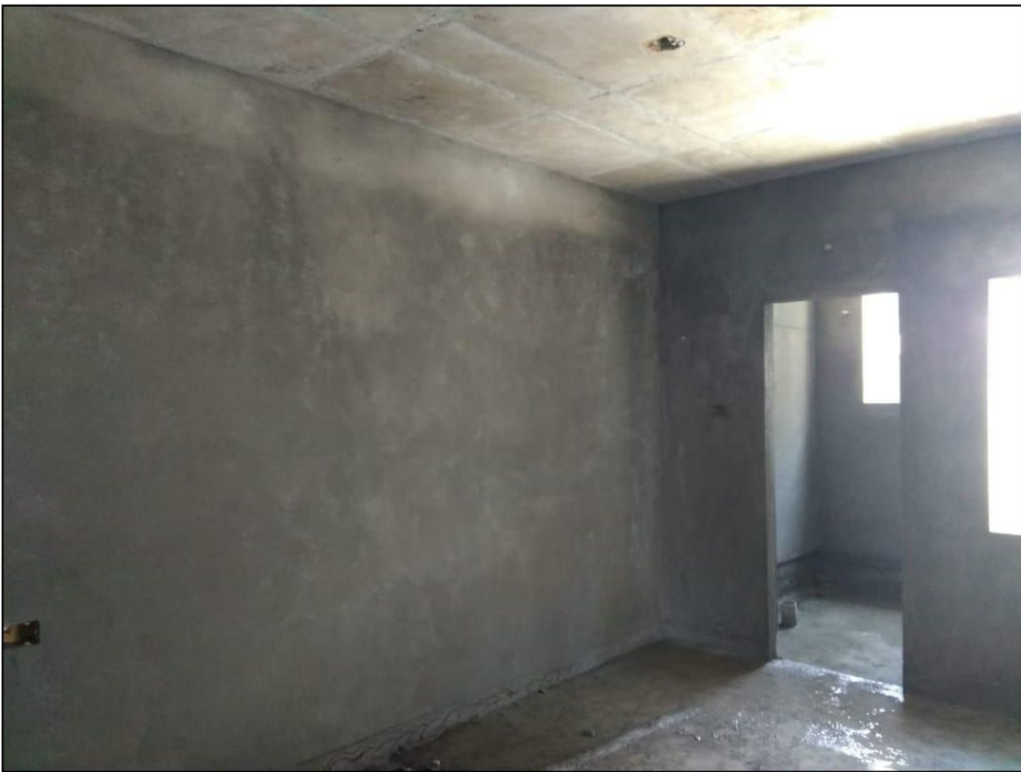
Internal plastering under progress
